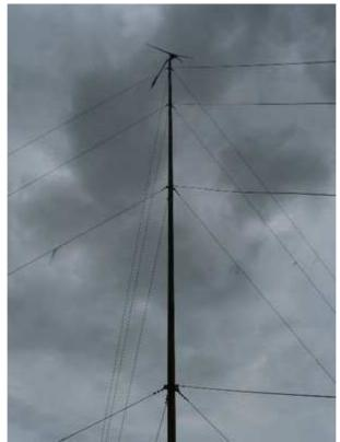
The 10 foot turbine looks tiny when observed from the ground, 80 feet below.
