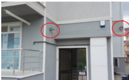
Fig. 20. An example of use of automatic lighting sensors a laboratory (Source: Provided by a participant laboratory)
