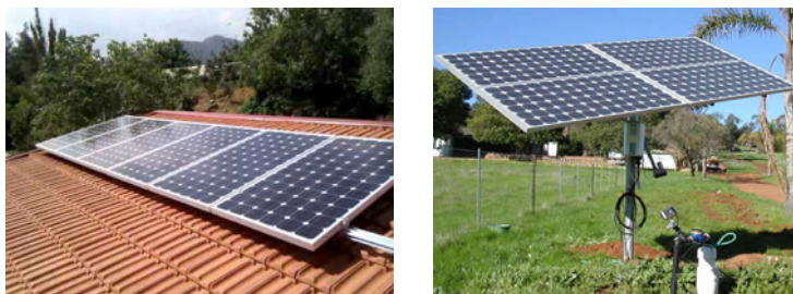
Fig. 22. Two examples of photovoltaic systems that may be utilised by laboratory facilities to produce renewable energy in countries where there is a high yearly amount of solar radiation (Source: http://www.k-energy.com.cy/en/services/photovoltaic-systems/18-k-energy/photovoltaics-and-solar-panels , www.arimec.eu )
