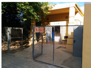
Fig. 14. Example of controlled access of a hazardous waste storage (Source: Provided by a participant laboratory)
