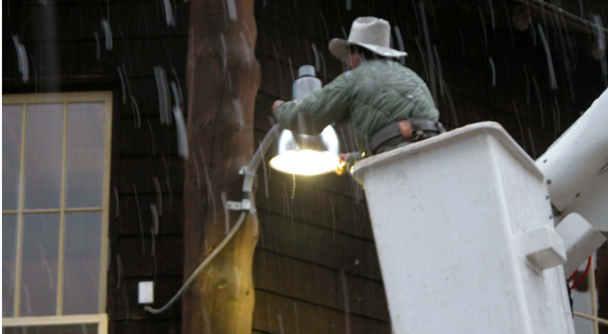
Figure 24. A full cutoff shield being installed on an existing light on the lodge at Yellowstone National Park. This previously unshielded light was visible across the lake and from the backcountry. Photograph by Travis Longcore.
