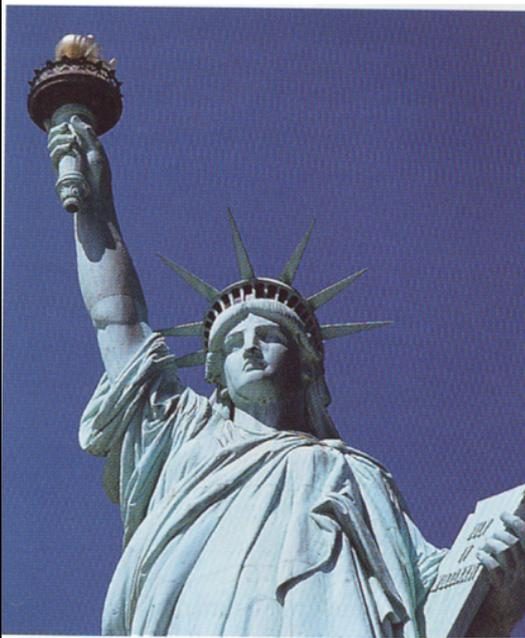
The outside of the Statue of Liberty is made from thin sheets of copper. Oxygen has oxidized the surface to copper(II) oxide. Further reaction with water and carbon dioxide has formed a blue-green coating of basic copper(II) carbonate of approximate formula  $\text{CuCO}_3 \cdot \text{Cu(OH)}_2$ .
