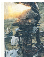
FIGURE 3.17 The dramatic reaction is being used here to produce molten iron that flows into a mold between rail casts, thereby welding the rails together. The thermite reaction has \Delta H^\circ = -847.6 kJ.
