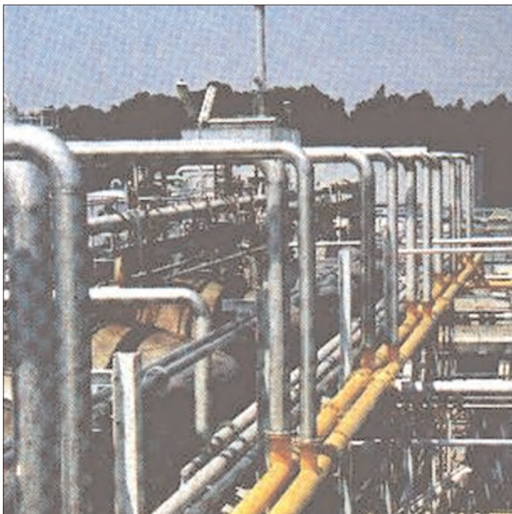
Figure 5. Closed Reactor: Connections Between Suspension Tanks and Gasometers (CIRES Archive).
