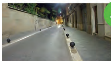
31W NW MSO H:6m, S:21m, Ancho 3m Ehmed 11lux, Uo =0.6 Ra 70 IRC: 70; Tc 4000K
